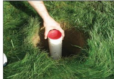
If you fail to push the sleeve into the gravel, it will allow the concrete to seal the hole and prevent water drainage.
