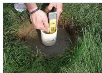
Remove the red cap to check the sleeve for plumb with a level in several locations. Install the red cap into the sleeve to prevent foreign objects from entering sleeve.
