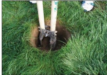
Dig a round Fence Post Size hole, 14" in diameter and 28" deep. A larger hole may be required for soft or sandy soil.
