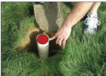
Use your "red cap" to cover the ground sleeve. Begin to shovel the concrete into the hole around the ground sleeve being careful not to disturb the sleeve position.
