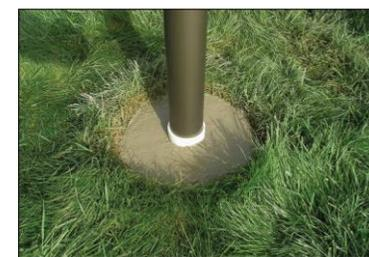
After a minimum of 24 hours of drying time, take off the red cap, place your flagpole into the hole.
