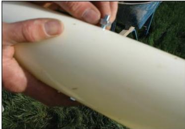
Install the stop bolt completely through the pre-drilled hole in the ground sleeve. Hand tighten only.
