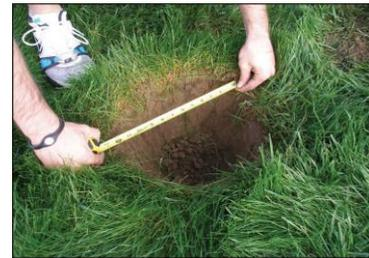
Be sure that your hole is at least the size stated in the previous step. Now shovel in 4-6" of gravel into the bottom of the hole. This will provide water drainage.
