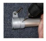
Attach the gold ball into the new top cap, slide the new stop ring and the new swivel ring over pole. Leave a small gap (1/8") between the top cap and stop ring which will allow the swivel ring to rotate freely around the flagpole.
