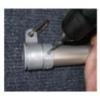
Attach the gold ball into the new top cap, slide the new stop ring and the new swivel ring over pole. Leave a small gap (1/8") between the top cap and stop ring which will allow the swivel ring to rotate freely around the flagpole.
